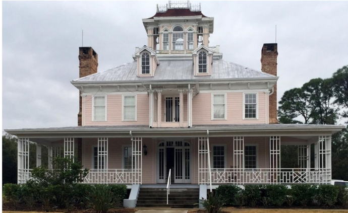
This 36-year-old house on Honore Avenue in Sarasota, with architecture inspired by the antebellum mansions of Eufaula, Alabama, could become a demonstration home operated by Sarasota's Universal Design Coalition. Or, it could be torn down. Fund-raising is under way. [COURTESY PHOTO]
